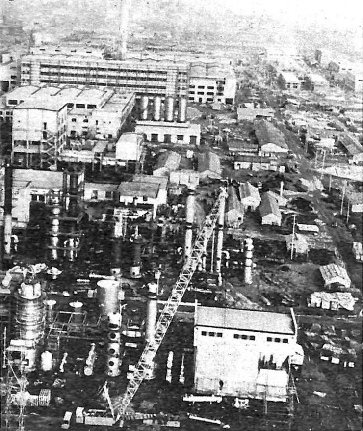
View of the Shanghai General Petrochemical Works.
